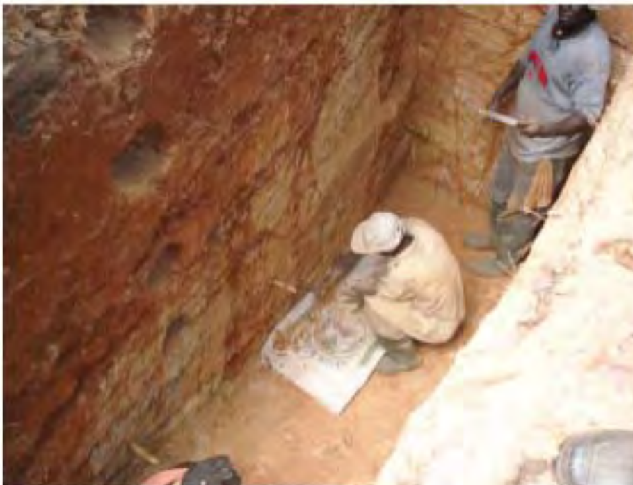
Figure 12.4: Channel Sampling in Trench at Apapam Concession
